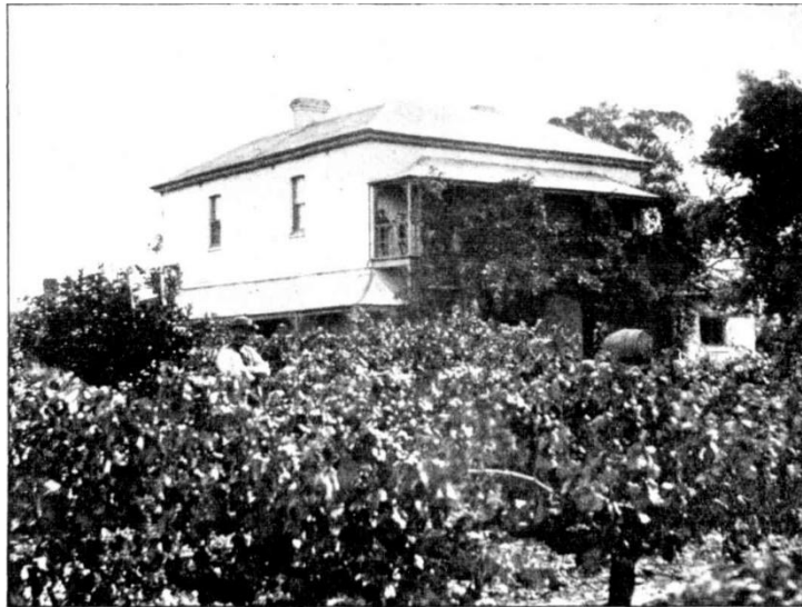
MR. HARDY'S RESIDENCE. WHICH NARROWLY ESCAPED DESTRUCTION.
