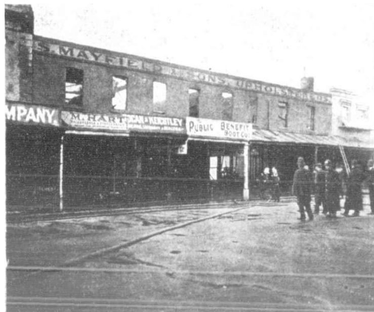
VIEW FROM RUNDLE STREET.
