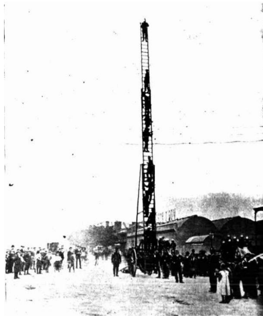
MANNING THE FIRE ESCAPE LADDER.
