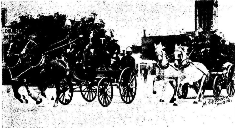
A TURN OUT.—GALLOPING TO THE SCENE OF THE FIRE.
